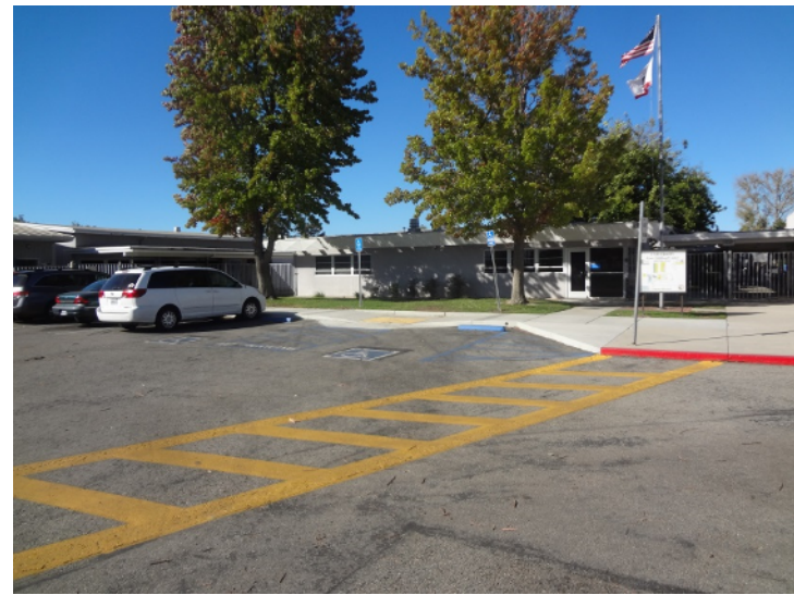
Photo -1 Building 1 Administration building and primary entry location to school.
