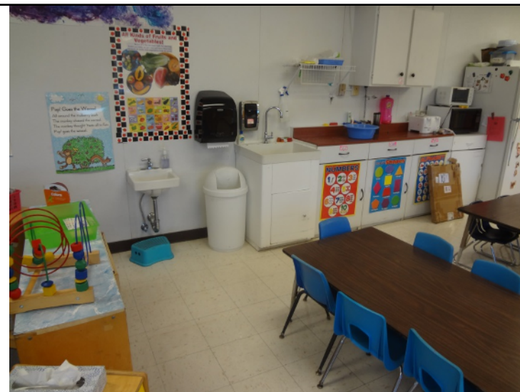
Photo -14 Building 7 Portable building interior, finishes are sufficient to the needs of the campus. Some buildings have accessible sinks.
