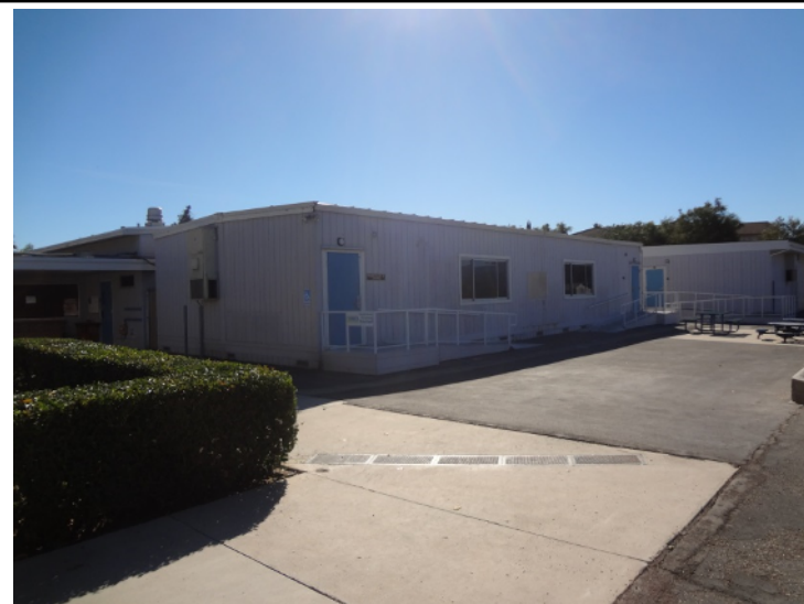
Photo -5 Building 7 Typical portable building on campus.
