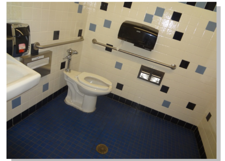
Photo -4 Most of the restrooms have received accessibility upgrades.
