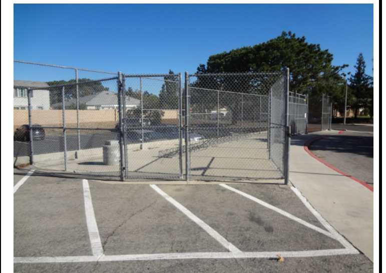
Photo -24 Parking Parking has been expanded over the years. The largest expansion is the conversion of the basketball courts to a parking lot. There are some accessibility issues in the parking lot.
