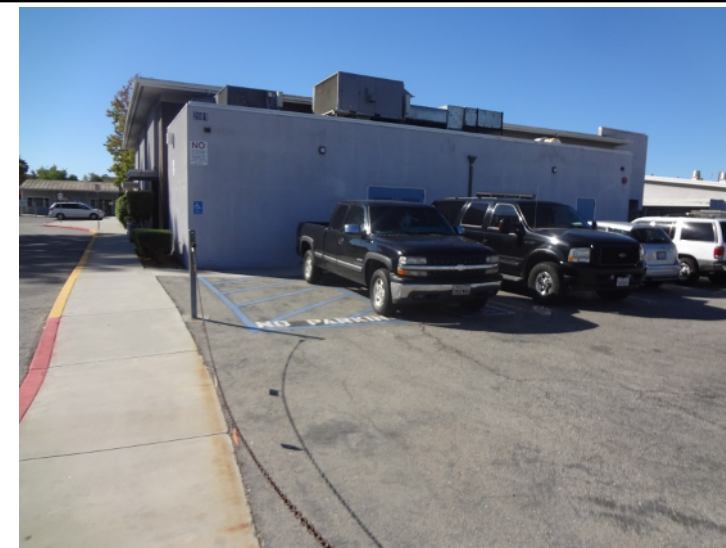
Photo -2 Building 1 Administration building looking toward the kindergarten classrooms. The original overhang over the administration building is deteriorating and should be removed.
