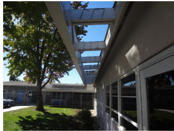
Photo -2 Building 1 Administration building looking toward the kindergarten classrooms. The original overhang over the administration building is deteriorating and should be removed.
